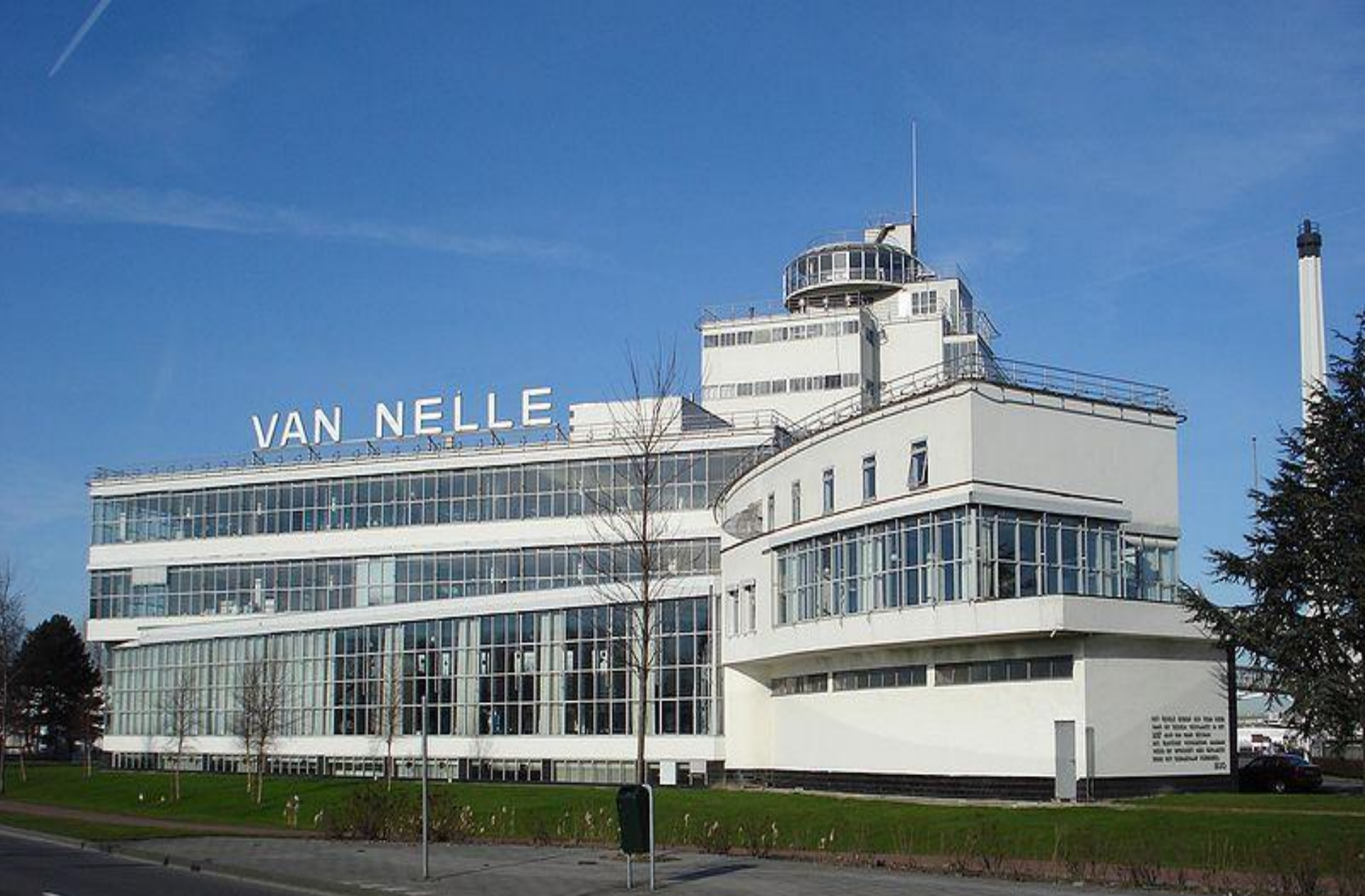
Van Nelle Factory in Rotterdam, The Netherlands by Leendert van der Vlugt and Mart Stam, 1925-1931
